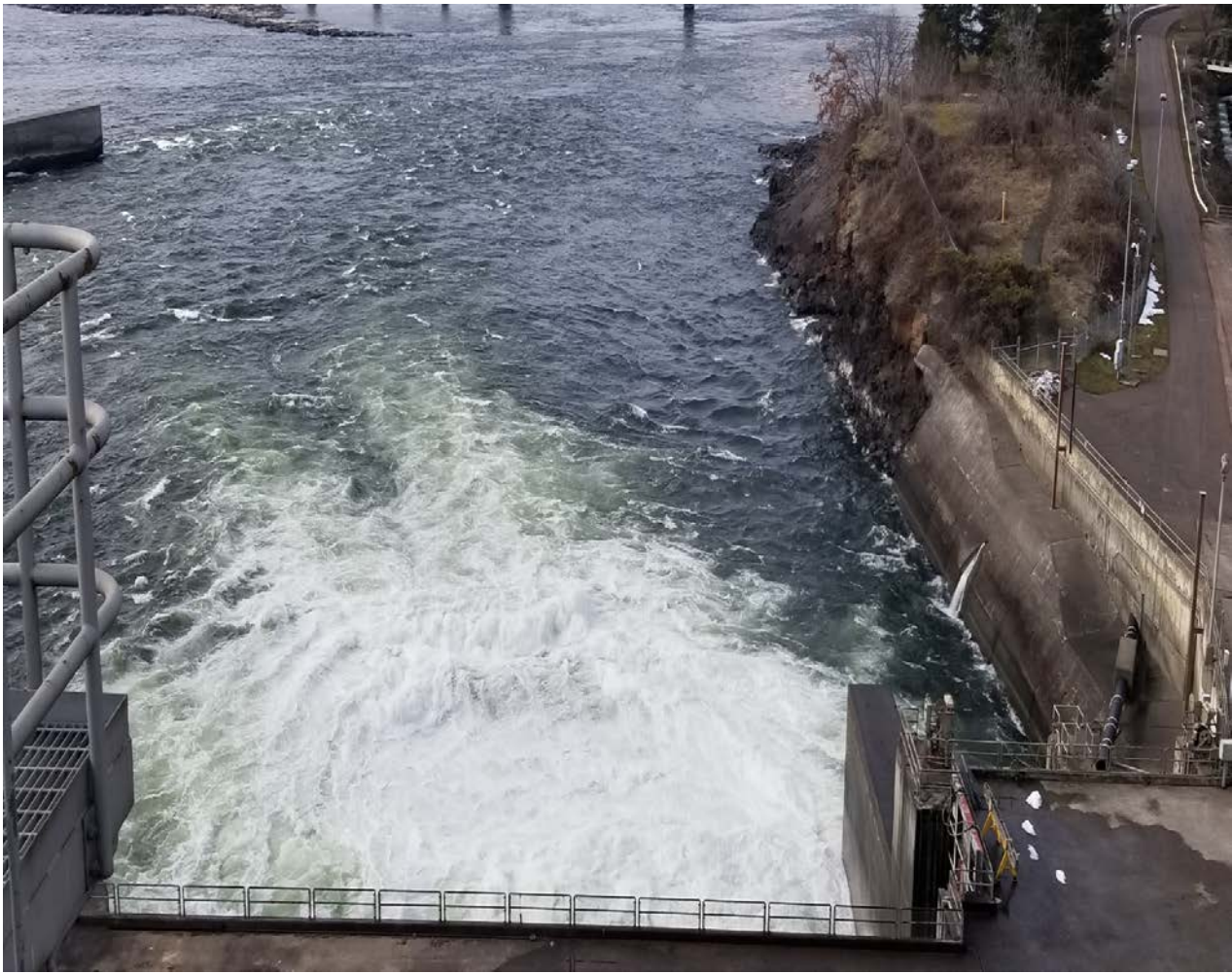
15kcfs through bays 1, 7 and 8 for attraction to north entrance due to no attractio flow for the east fishway
